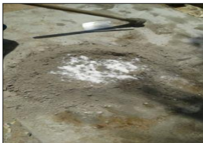
Figure. 9 At The Stage Of Chemicals Addition ( \text{NaOH} & \text{Na}_2\text{SiO}_3 )
